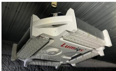
Installation of LED lightings with motion detected sensor
