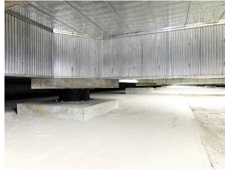
Seismic isolators
