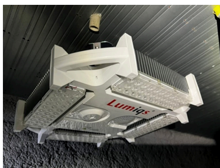
Installation of LED lightings with motion detected sensor
