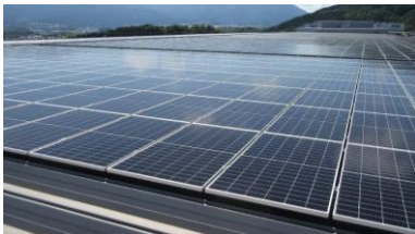
Installation of solar panels
