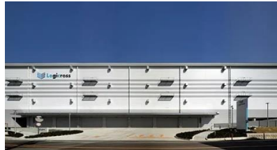
Installation of sandwich panels for exterior walls
