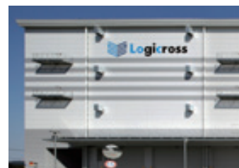
Insulated sandwich panels for exterior walls
