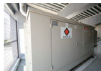
Installation of private power generators
