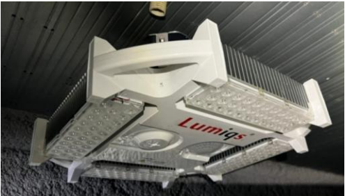
Installation of LED lightings with motion detected sensor
