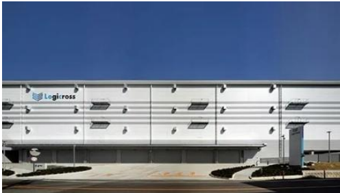
Installation of sandwich panels for exterior walls
