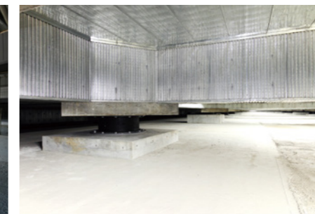
Seismic isolators
