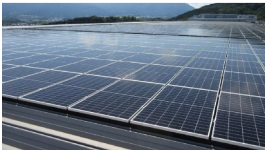
Installation of solar panels
