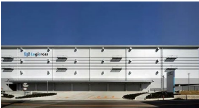
Installation of sandwich panels for exterior walls
