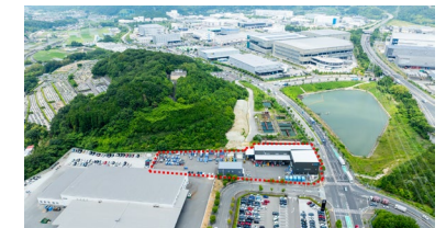
MJ Industrial Park Kobe-Nishi
