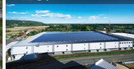
MJ Logipark Tsuchiura 1
