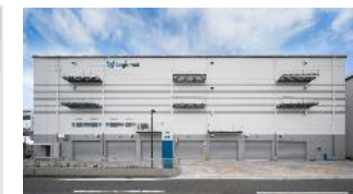
Logicross Yokohama Kohoku
