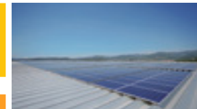
Installation of solar panels
