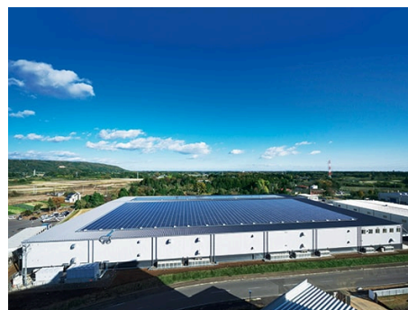
MJ Logipark Tsuchiura 1
