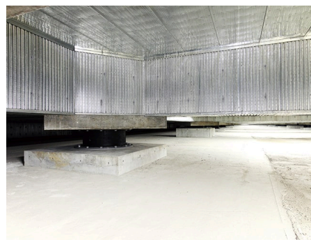
Seismic isolators
