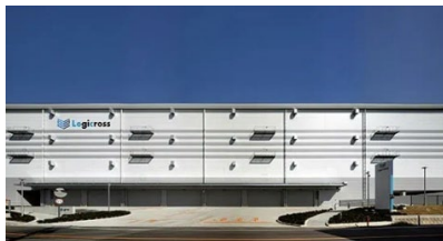
Installation of sandwich panels for exterior walls
