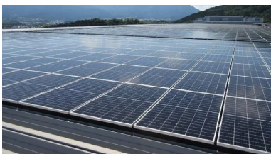
Installation of solar panels
