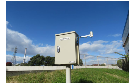
Irrigation system with rain sensor
