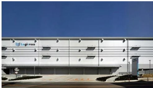
Installation of sandwich panels for exterior walls
