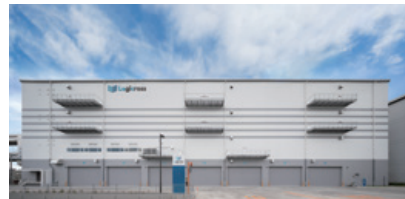
Logicross Yokohama Kohoku
