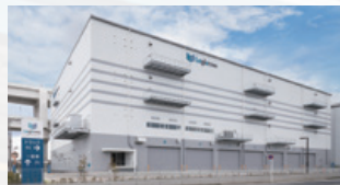
Logicross Yokohama Kohoku
