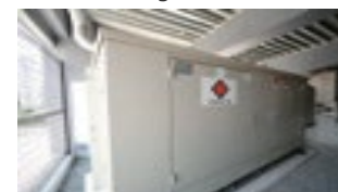
Installation of emergency power generators
