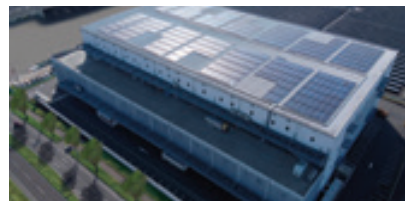
MJ Logipark Sendai 1 Acquisition price 7,388 million yen Occupancy rate 100.0%
