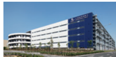
LOGIPORT Kawasaki Bay (co-beneficiary interests 45%) Acquisition price 36,000 million yen Occupancy rate 99.9% CASBEE A Rank for New Construction
