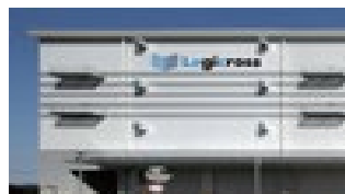
Insulated sandwich panels for exterior walls
