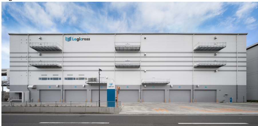
Logicross Yokohama Kohoku
