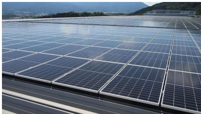
Installation of solar panels
